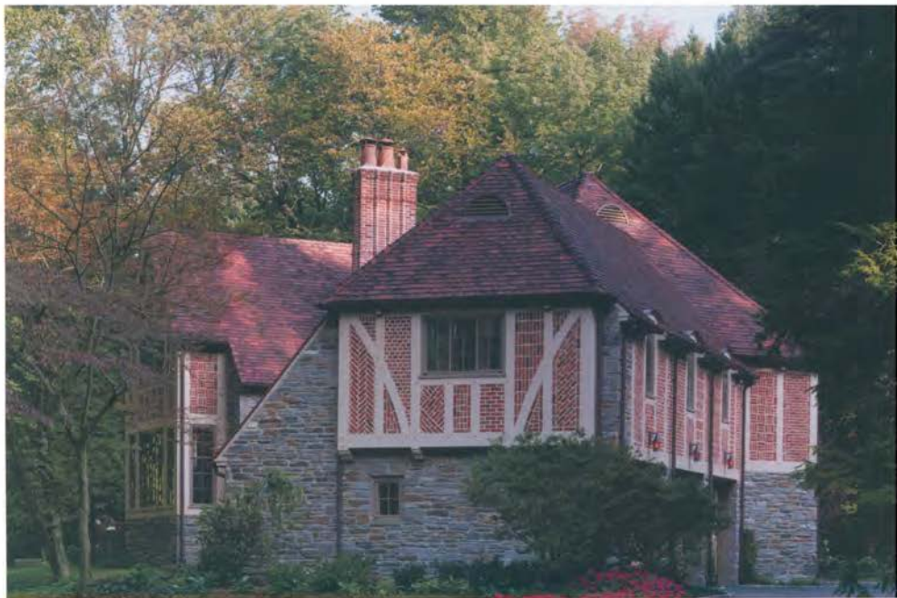
The oblique siting of the new garage hides the garage doors — by Artisan Custom Doorworks of Bristol, PA — from immediate view and opens the approach into the new entrance courtyard. The ironwood trees at the corner of the garage were protected during construction and give a sense of scale to the landscape; the azaleas were removed and replanted after construction.
