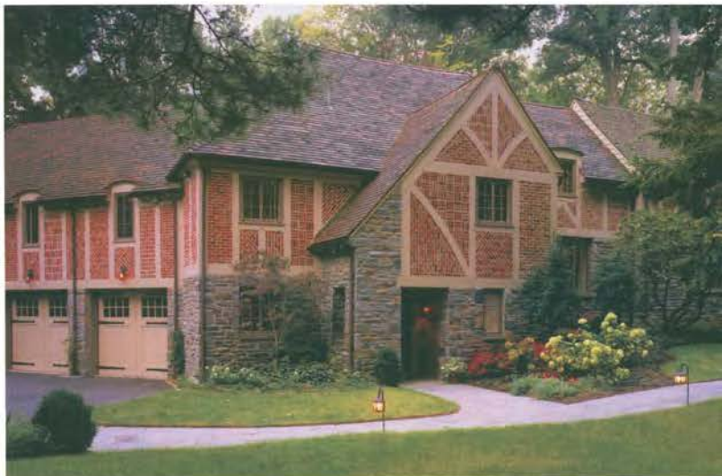
Peter Zimmerman Architects added 3,000 sq.-ft. to a ca. 1935 Tudor-influenced residence in Bryn Mawr, PA, in order to accommodate a growing family. The addition comprised a family entry, three-car garage, family dining room and three new bedrooms and baths.
